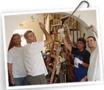
Employees paint homes of elderly people in Rosh Ha'ayin before Passover
